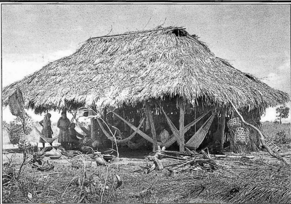
PLATE 11 NORTHERN SAVANNAH, 1949 UNFINISHED MAKUSHI HOUSE (Note thatching palm in foreground)
