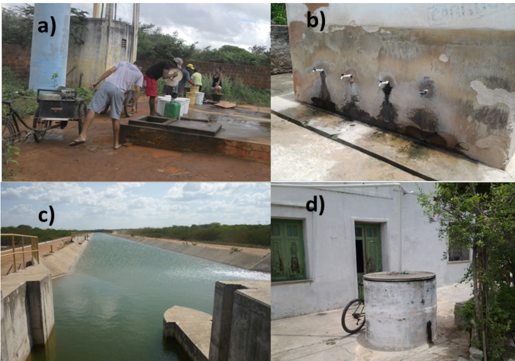
Figure 2 – Identification of some of the sources of water in the Cristais community: a) community cistern; b) public fountain; c) river basin integration canal; d) rainwater reservoir
