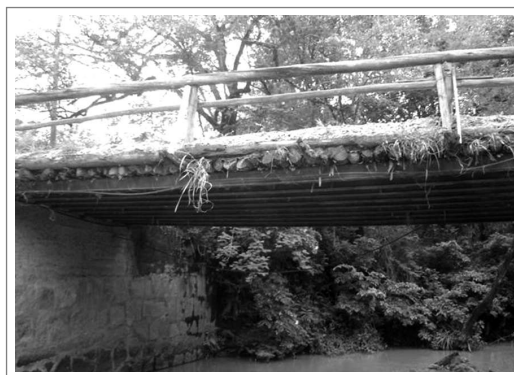
Figura 2. Vista general del puente Figure 2. Bridge overview
