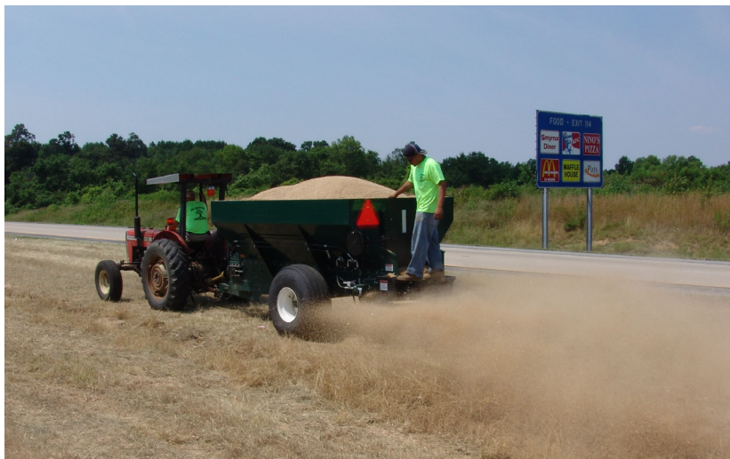
Figure 3. Sawdust is successfully used as a medium for distributing seed on a highway median.
