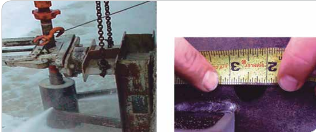
Fig 1. Cutting performed on 5 1/2 in cemented casing.
