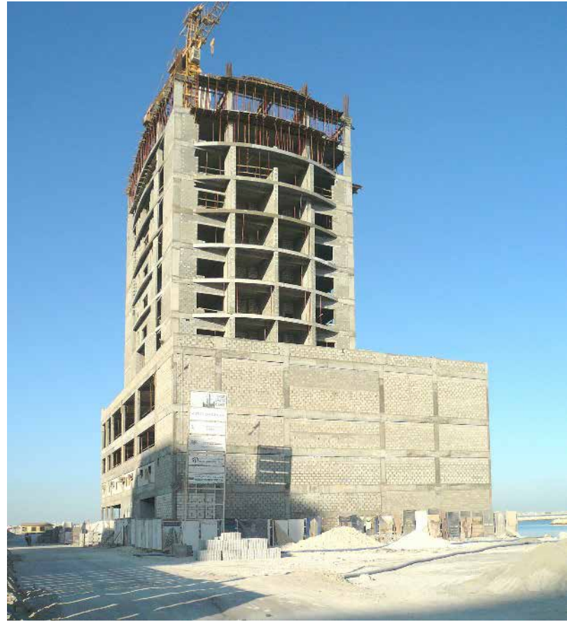
Figure 8. Integrated multi-story car park at a construction site of a residential high-rise in Manama's Juffair district. © Wiedmann.
