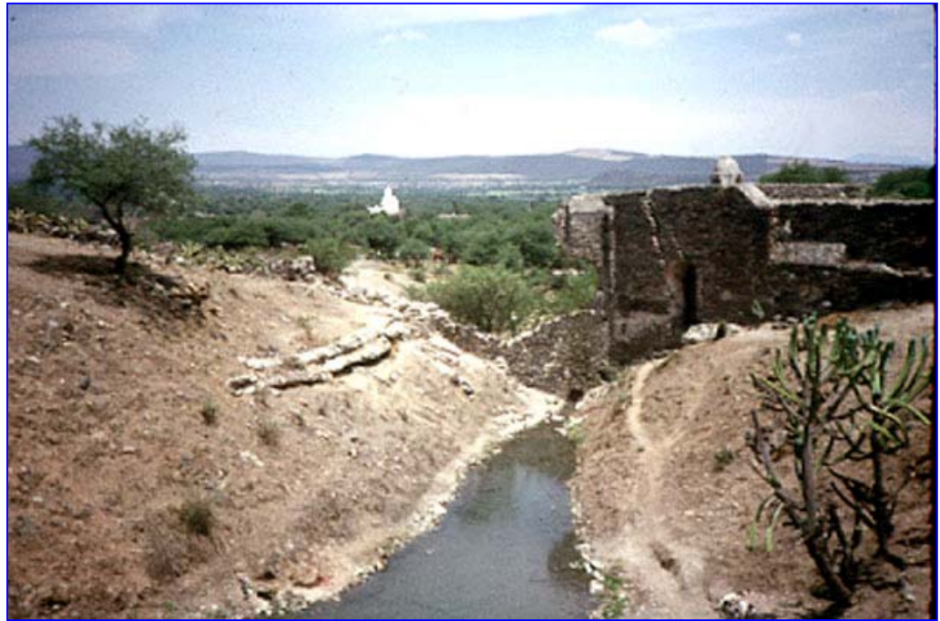
Fig. 9. Thermal waters from this spring flow into the aqueduct that goes down to the spa. The church dome in the spa complex is visible in the distance
