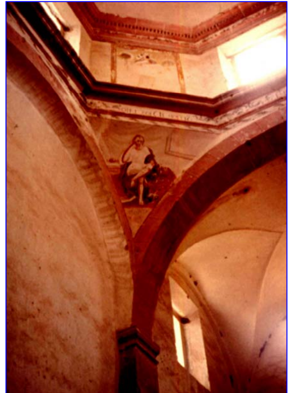
Fig. 4. Niches by the arches around the church dome are decorated with delicate paintings of the apostles at rest, some washing their feet, suggesting the religious nature of healing experiences in the spa's thermal waters.
